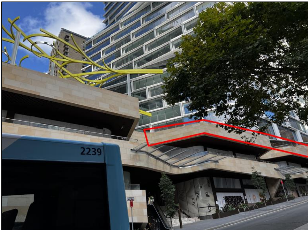
Figure 2: Site viewed from the Young Street frontage, including the location of the proposed outdoor seating area
